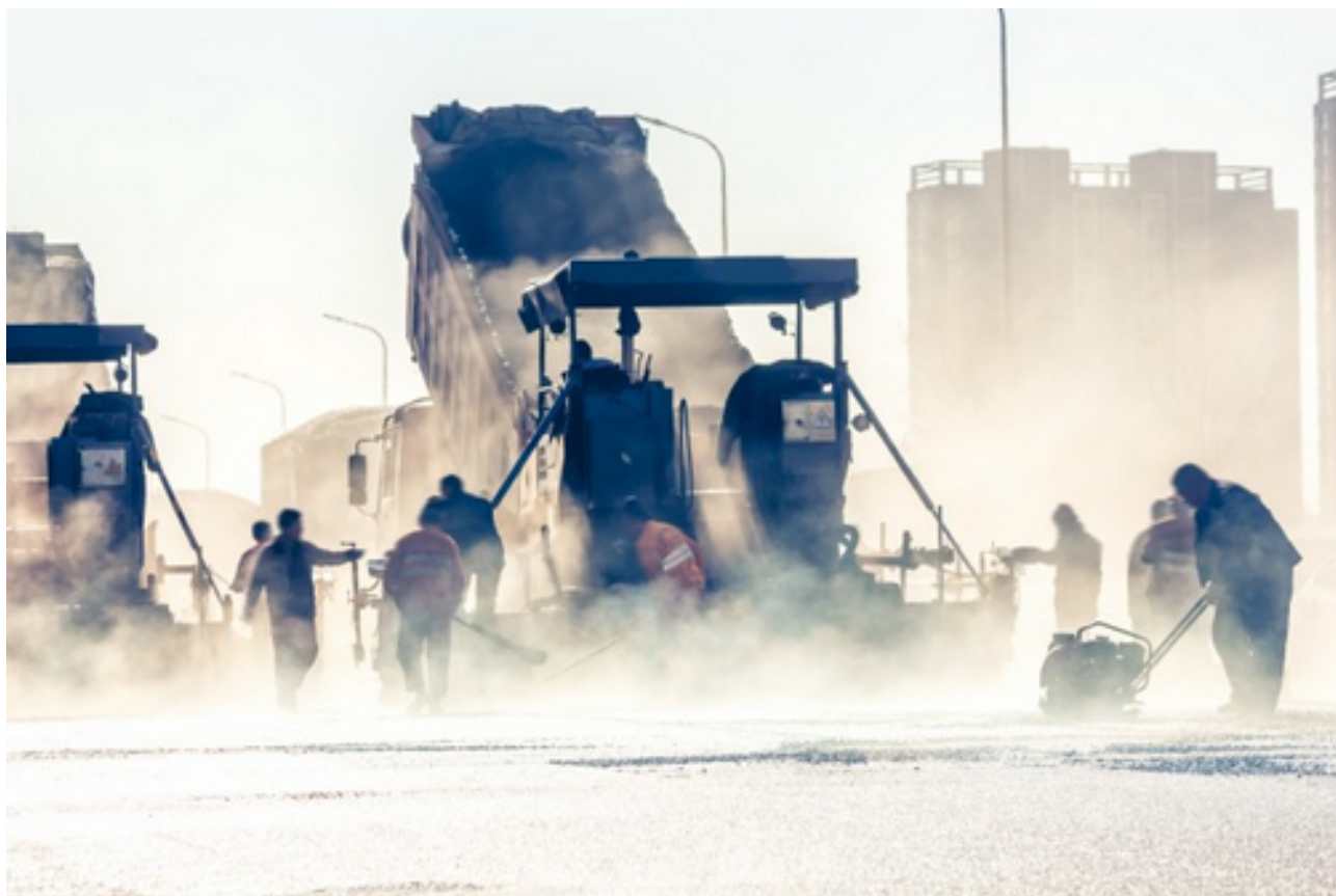
Building Roads (Photo credit: user 06photo via Shutterstock)
